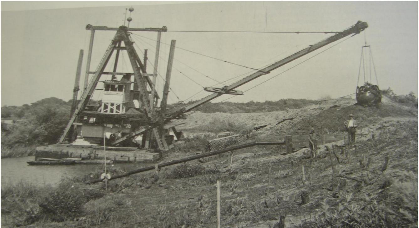
**Figure 1.** Construction of a Levee by Clamshell Dredging in California around 1910
